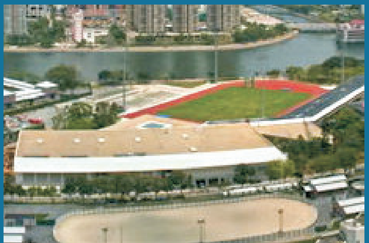
Hong Kong Sports Institute - Ventilation System
