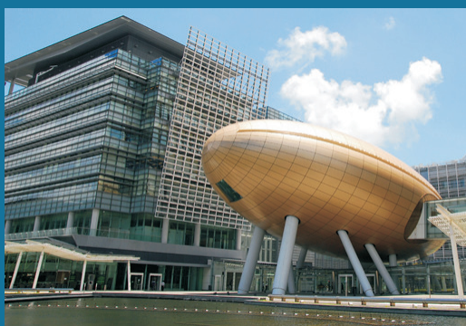
Hong Kong Science Park Phase2 C Zone Ventilation System
