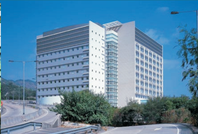
Public Health Laboratory Centre- Ventilation System
