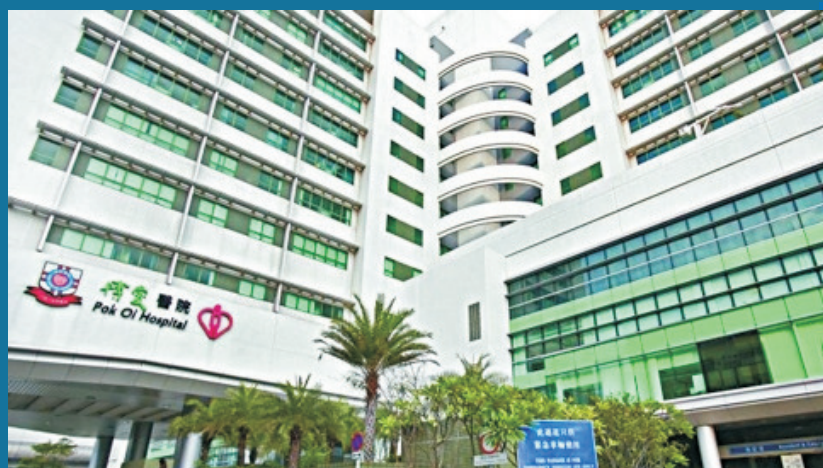
Pok Oi Hospital- Ventilation System
