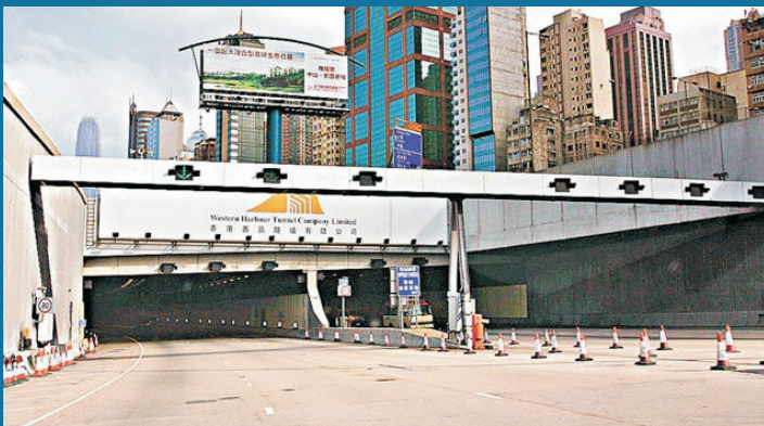
Western Harbour Tunnel Ventilation System
