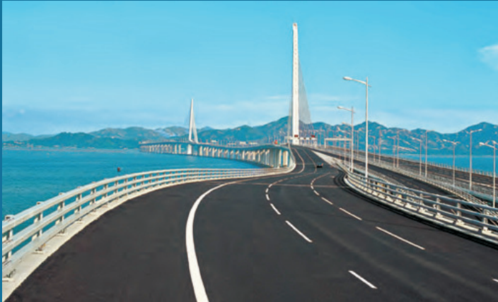
Cable Placket Supply Hong Kong-Shenzhen Western Corridor
