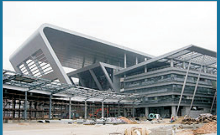
Hong Kong-Shenzhen Western Corridor Building Ventilation System
