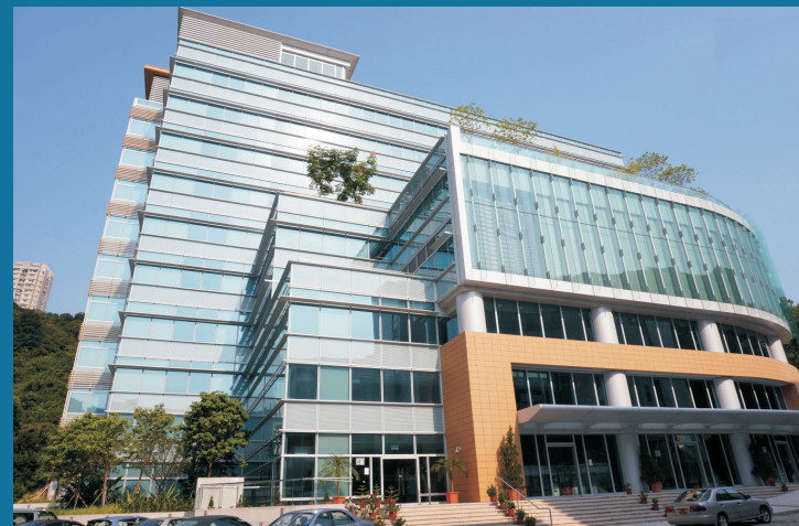
Heng Seng Management College Block D - Chill Ceiling Supply
