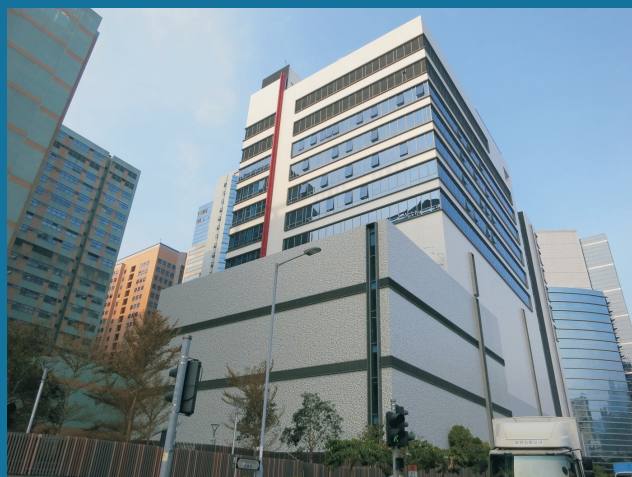
HSBC Data Centre at Shek Mun Ventilation System
