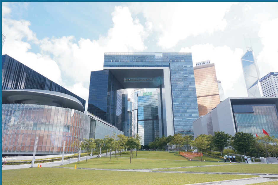
Government Headquarter- Ventilation System
