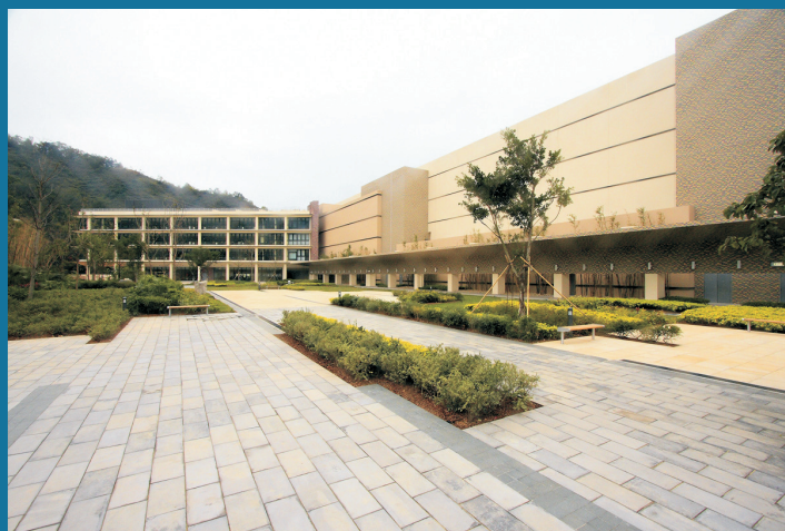
HSBC Data Centre at TKO Ventilation System
