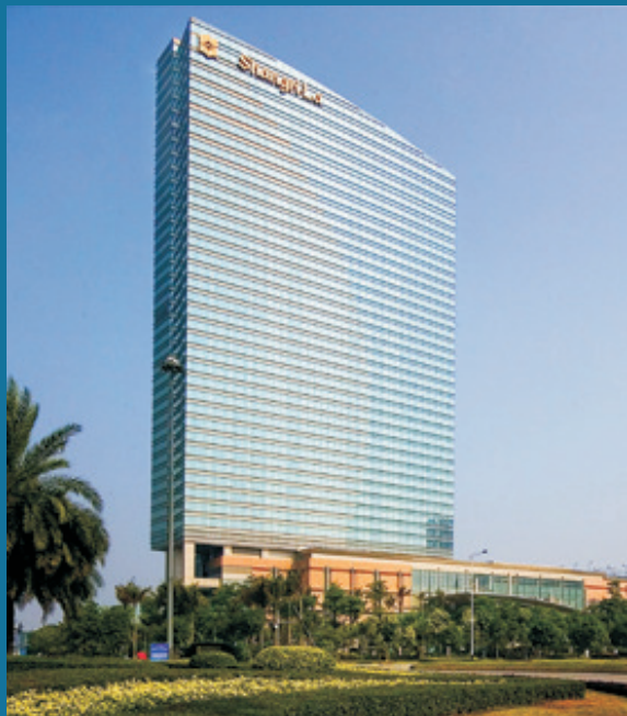
Shangri-La Hotel, Guangzhou Ventilation System.
