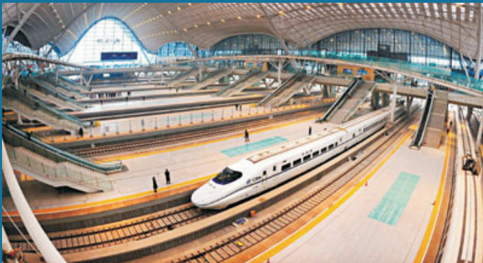
Guangzhou Shenzhen Hong Kong Express Rail Link Ventilation System
