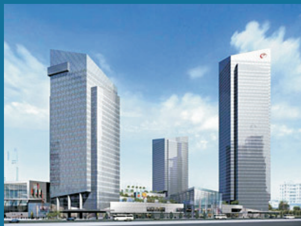
Taikoo Hui, Guangzhou, Tianhe Ventilation System
